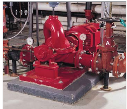
High Pressure Two-Stage DMD Fire Pump.
