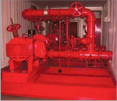
Completed housed unit.
